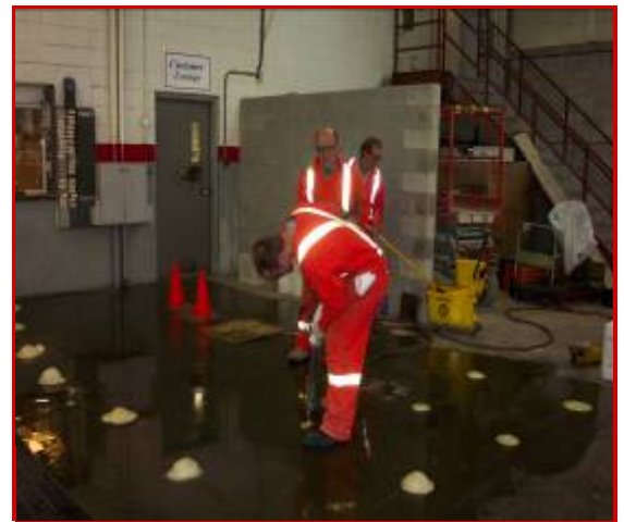
RIGID GROUT is a cost effective solution to fill voids beneath concrete slabs.
