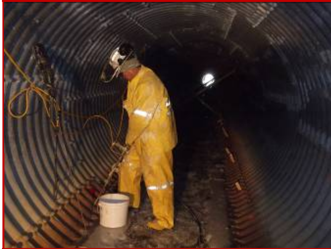
RIGID GROUT is used to fill voids in culverts beneath an airport runway. Repairs were required to prevent settlement.
