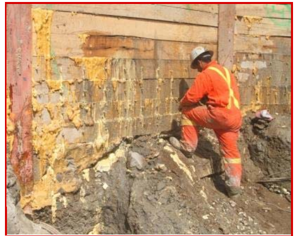
Multiurethanes ULTRAFINE RESIN is used to stabilize soil seepages beneath shored excavations.
