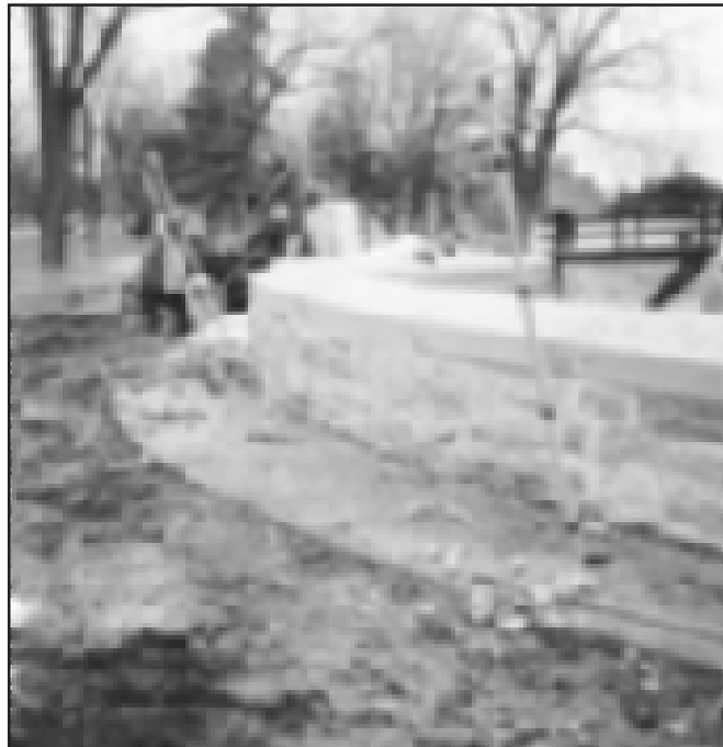
Low viscosity polyurethane resins such as ULTRAFINE are used in conjunction with sleeve pipe systems for the stabilization of water-bearing soils beneath historical structures
