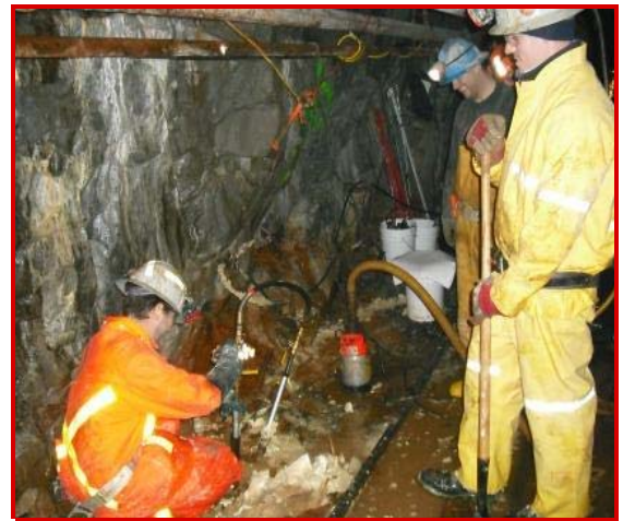
UNIVERSAL RESIN is used to stop water inflow problems for tunneling contractors.
