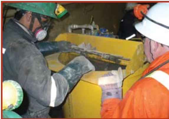
Pan American Silver, Huaron Project, Peru Cement grouts were used to reduce high volume water inflows through fractured and water-bearing ground conditions prior to shaft construction using conventional sinking methods.
