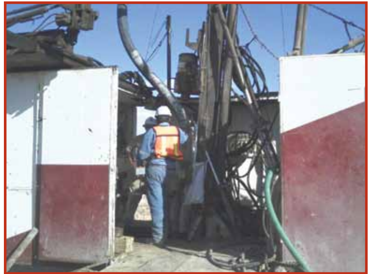
Excellon Resources, Platosa Mine, Mexico Deep hole drilling and high-volume cement grouting operations were used to seal water-bearing rock formations and successfully recover a flooded underground silver mine.
