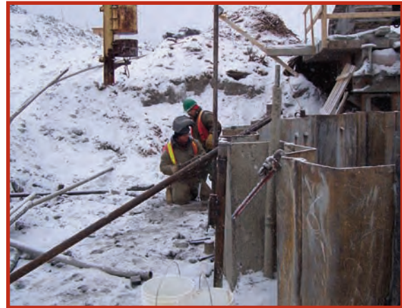
Agnico-Eagle, Goldex, Quebec Construction of a shaft collar through quick sand was overcome using a systematic engineered grout plan. The plan specified strategic placement of grout pipes as well as appropriate cement grout mixture for this unique application.
