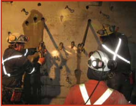
Hudbay Minerals, 777 Mine, Manitoba Specialized grouting equipment and technical support was used in the construction of two high-pressure concrete bulkheads.
