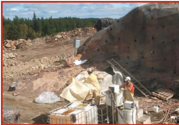
FNX Mining, Podolsky Mine, Ontario Pre-grouting of raise bore holes was completed using microfine cement grouts, equipment and technical support.
