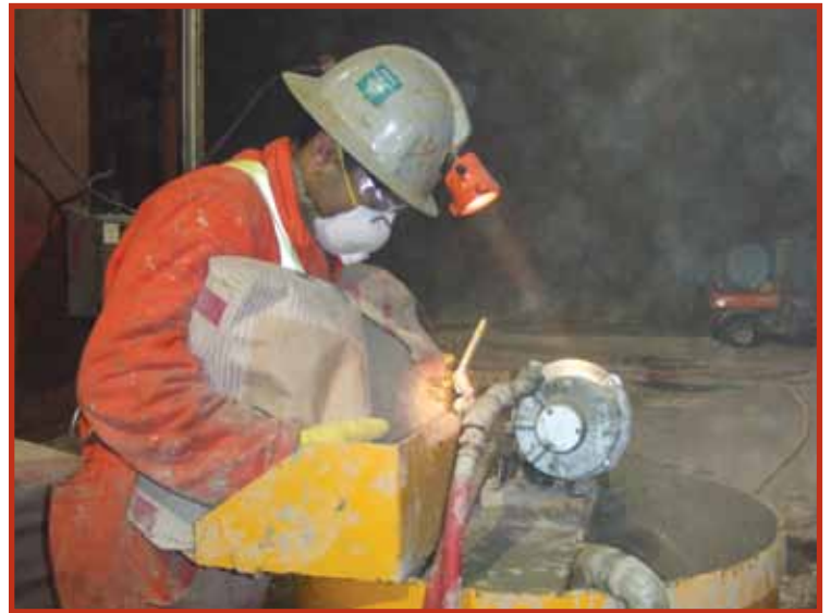
Sifto Salt, Goderich Mine, Ontario Chemical grout, applied as spray foam, was used to seal a five meter high by eight meter wide underground ventilation bulkhead. A layer of cement grout (in the form of spray foam) was applied over top for fire protection purposes.
