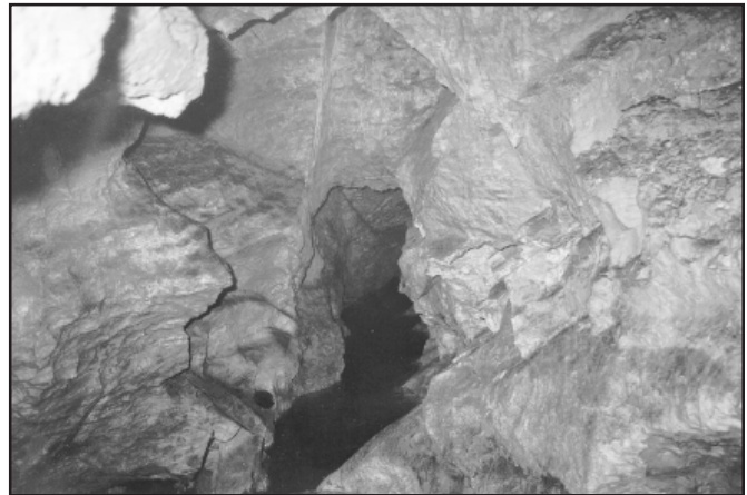
Cement grouts are used to seal underground cavities such as this underground solution cavern that was discovered at an underground limestone mine where flowing water had eroded weak stone layers
