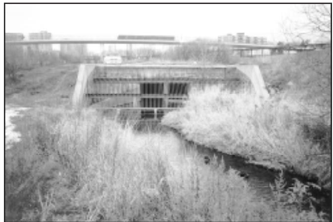
Storm sewer and diversion tunnel outfalls connecting directly with wetlands and fish spawning streams are sealed using MULTIURETHANES products to the satisfaction of local environmental authorities
