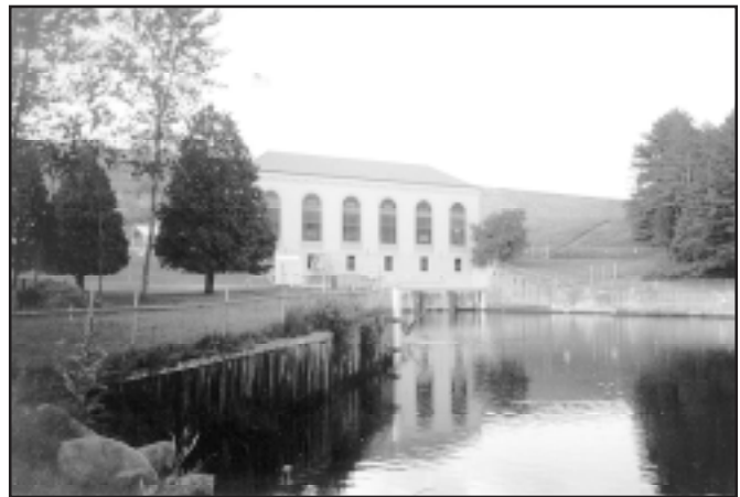
The tailrace of this hydro electric generating plant is typical of major project sites where MULTIURETHANES products are successfully applied without serious environmental consequences
