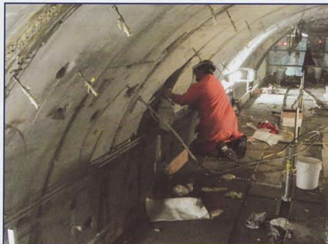
Multiurethanes Universal Resin is used to stabilize soil and cut off water flowing from leaking joints of precast tunnel segments.
